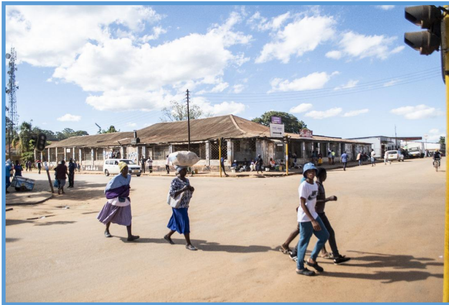
Figure 18: State of Some Buildings Old Chipinge Hotel
