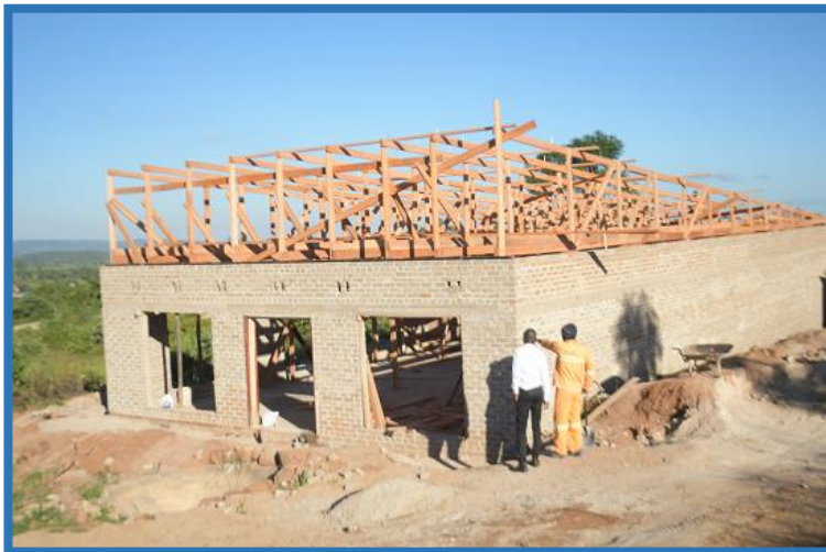
Figure 55: Shop under Construction at a New Shopping Centre
