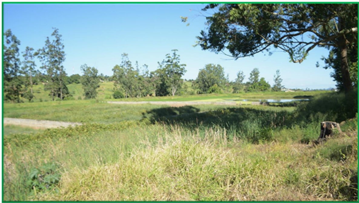
Figure 44: Sewer Treatment Plant
